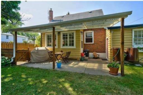
Concrete Patio off Sun Room
